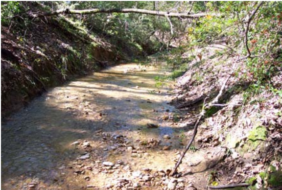
Figure 1. Gully after rainfall. Note level, rocky floor.
